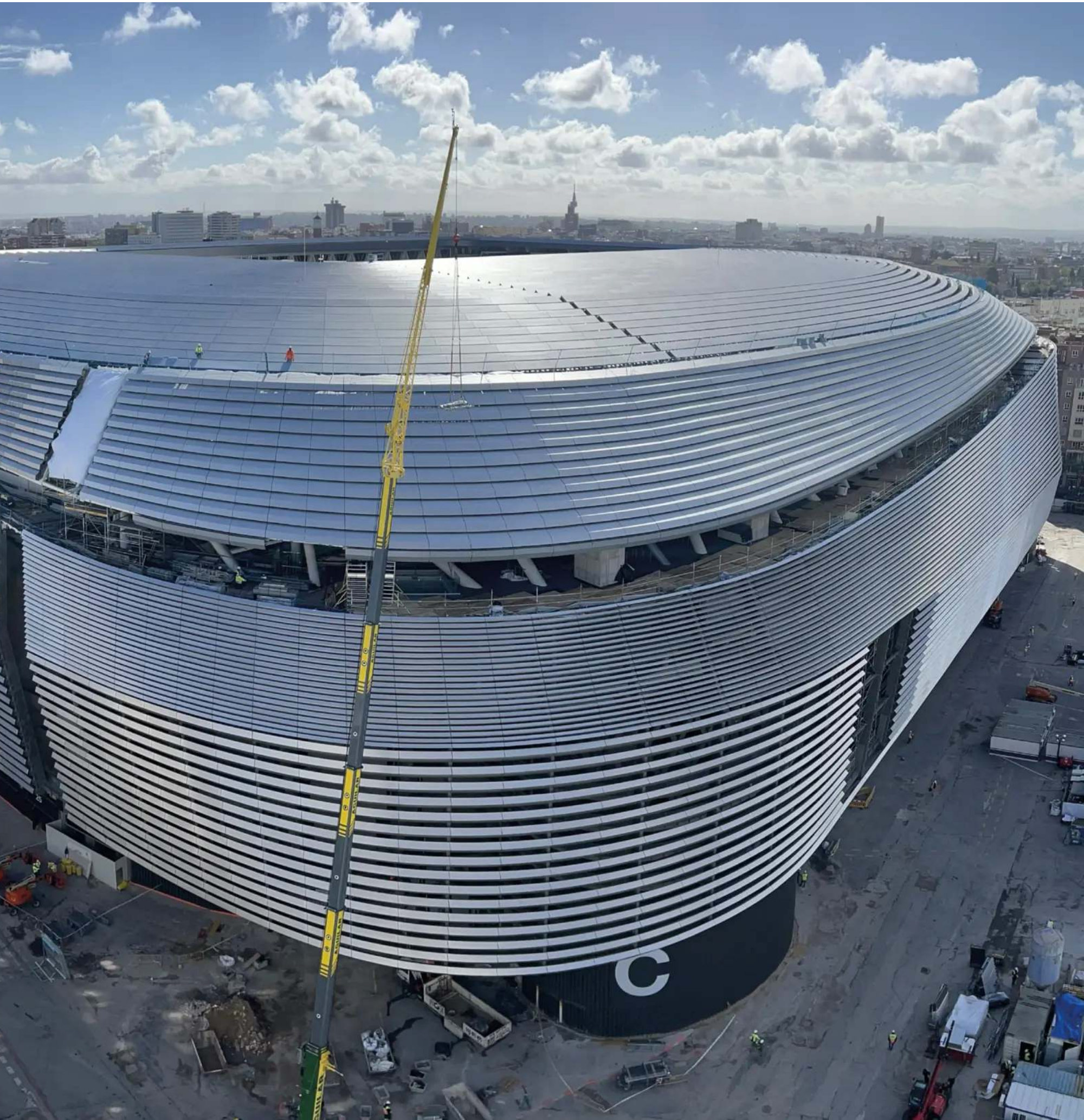
Construction of the emblematic Santiago Bernabéu Stadium.
