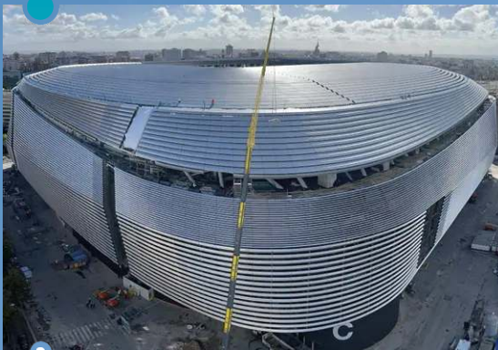
The Santiago Bernabéu, built by FCC Construcción, chosen as the best stadium in the world by the World Football Summit
